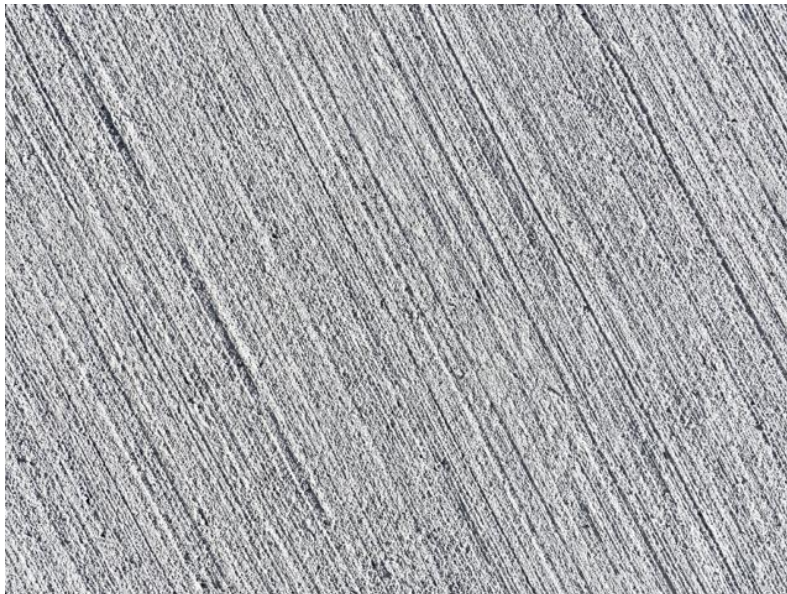
Figure 10 - Dalle béton balayée
