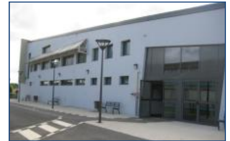
Salle modulable Gymnase
